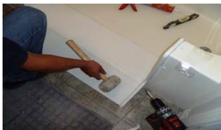
Setting the non-skid threshold:
