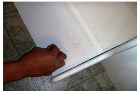
Plugging the screw hole
