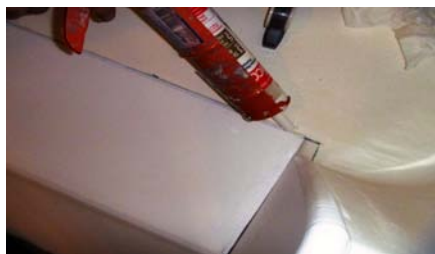
Caulking the tri-seal:
